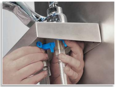
Faucet installations just got a whole lot easier! Sinchnuts are a new kind of nut. They're hinged, which allows you to wrap them around the faucet shanks at a high position. No more endless turning like with brass nuts. It also allows you to connect the supply lines *before* you mount your faucet. No more crawling under the sink. Faucet installations are a cinch with Sinchnut!
